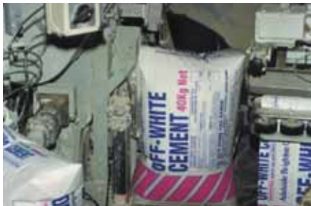
Cement Filling Station
